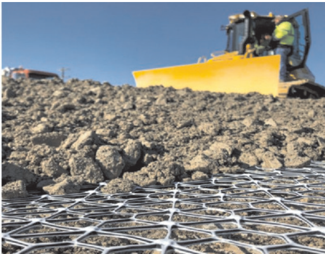
Fig. 19: Geogrid in subgrade reinforcement
