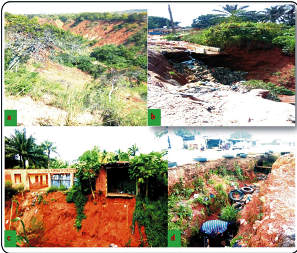
Fig. 1: Gully erosion ravaging the area
