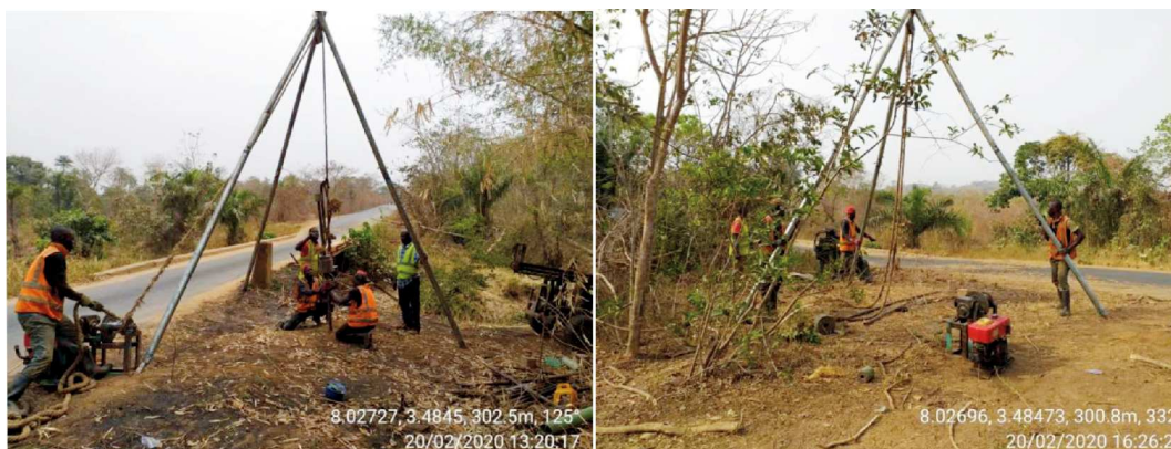
Fig. 2: Field investigation equipment set-up at Okeho and Iseyin abutments
