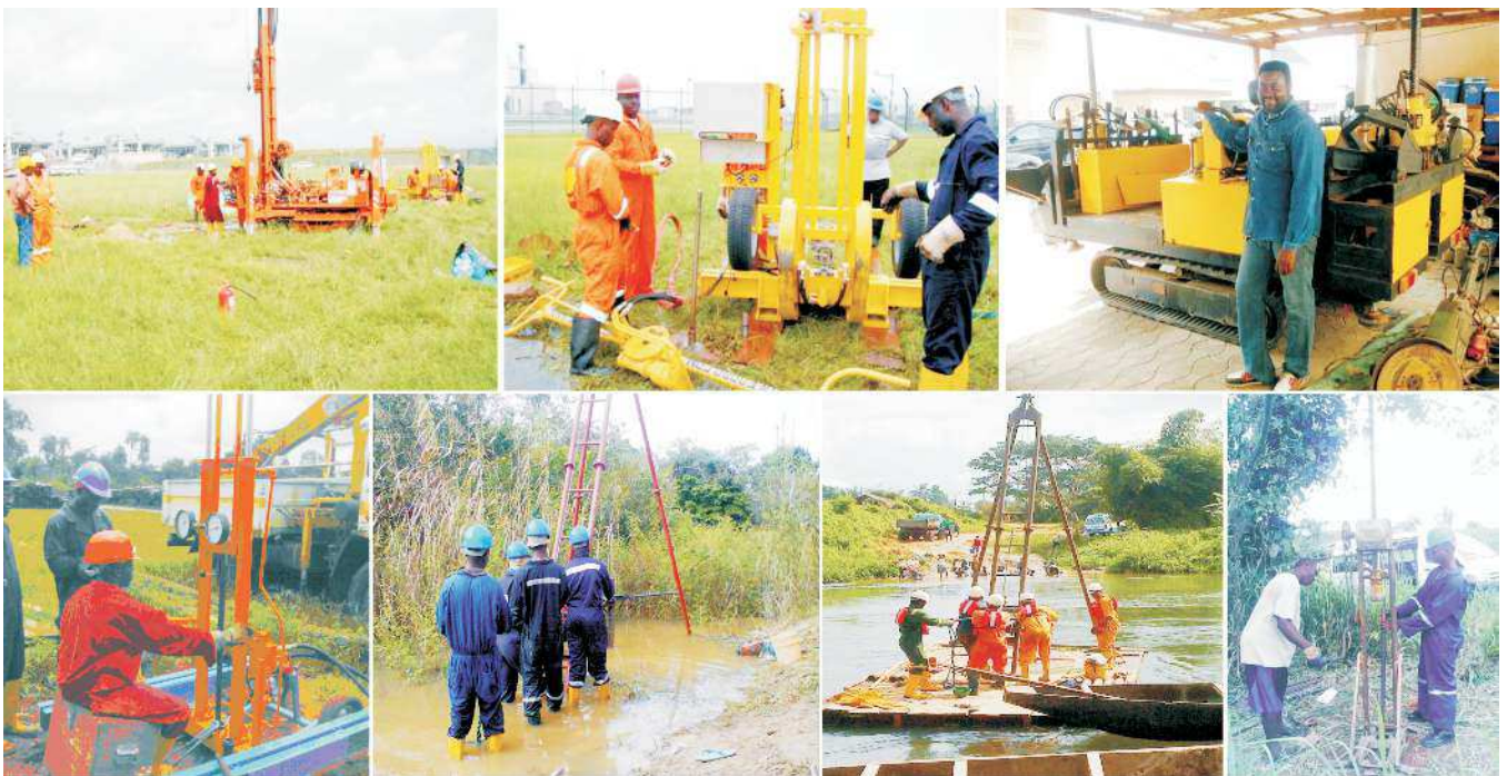
Fig. 2: Some equipment used for soil investigation and site conditions for work
