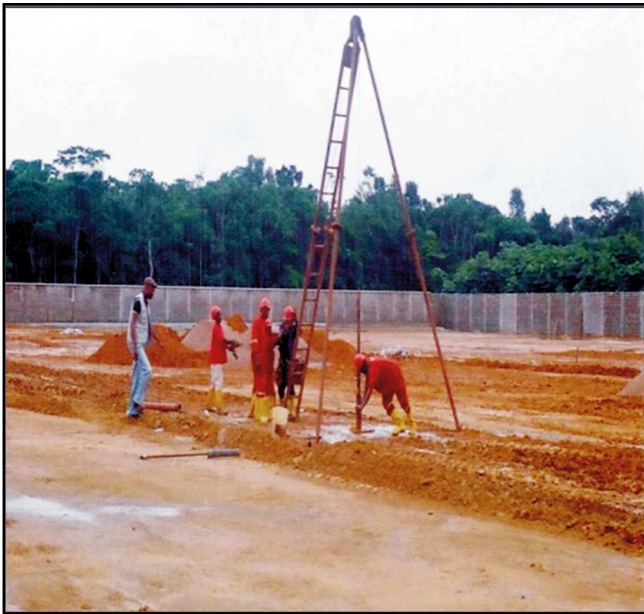
Fig. 2: Percussion Rig drilling in Process at the project site
