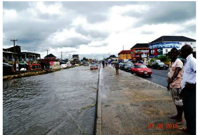
PLATE 3: Flooded UNIPORT bound lane of EAST-WEST HIGHWAY at Nkpolu Road Junction
