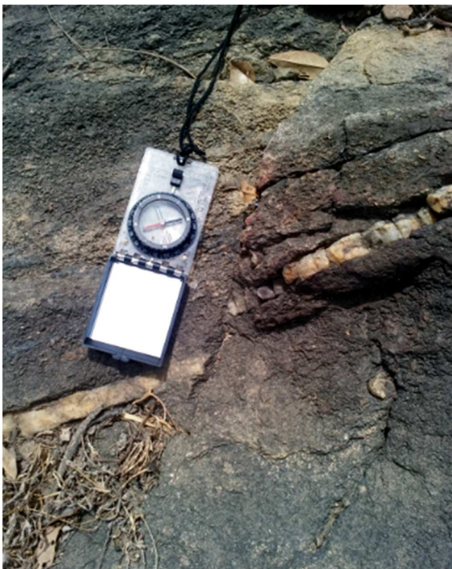
Plate III: A sinistral fault 09 °38' 37", 06° 37' 0"
