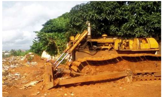
Plate 9: ASWAMA bulldozer used to clear & push solid waste into landfill
