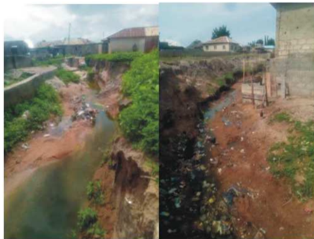
Plate 6: (left), one side drainage was cast to prevent soil erosion in Sauka (9° 35'28"N, 6° 31' 18" E)
