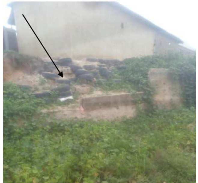
Plate 4: Tyres were used to stop soil erosion at Kpankungu (09° 35' 44" N, 006° 31' 25" E).
