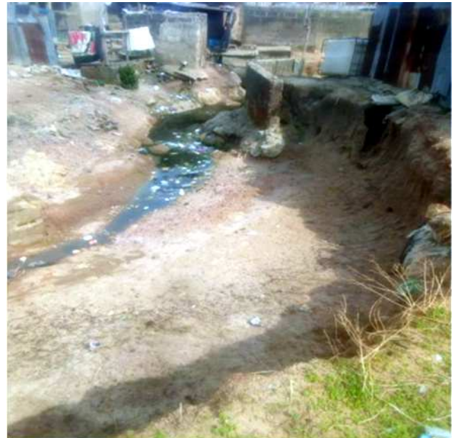
Plate 8: Building destroyed by soil erosion in Tunga (9° 34'29"N, 6° 34' 1" E)
