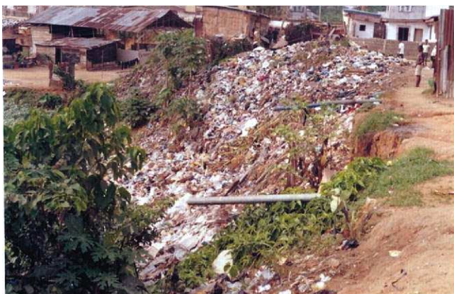
Plate 1: Sewage pipes channeled directly into the Borrow Pit
