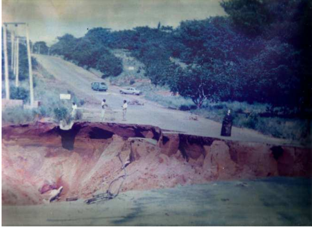
Fig. 6(a): Umunnkwu erosion site along Uturu - Isuikwato Road, 1996
