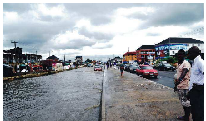
Fig. 5(c): Flooded UNIPORT bound lane of EAST-WEST HIGHWAY at Nkpolu Road Junction
