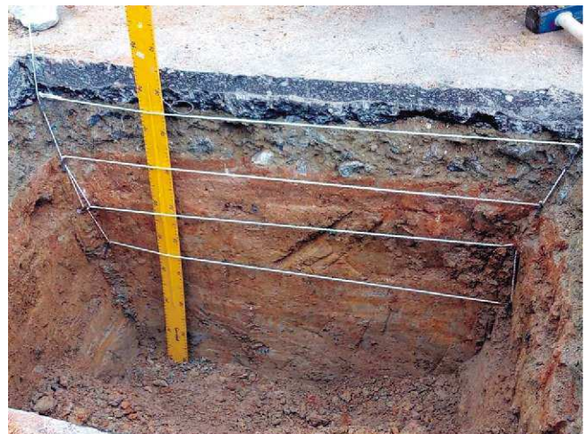
Appendix D: Picture plate for Trial pit lining with sampling depth
