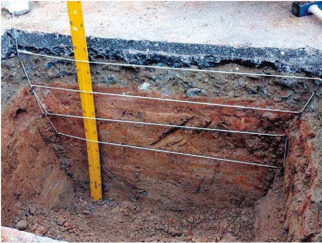
Appendix A: Picture plate for Trial pit
