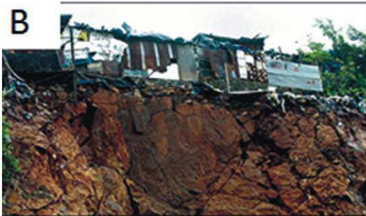
Houses stand on the edge of a landslide in the Seli Nala suburb of Mumbai. Ref: www.chinadaily.com
