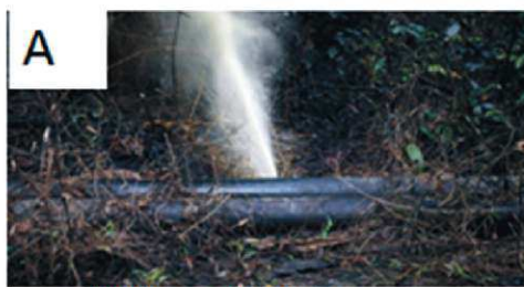
A Oil pipeline spews oil after leakage Ref: Akitunde Akinleye/Reuters
