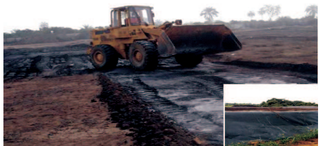
Plate 5: Ex-situ Landfarming/Tilling of Hydrocarbon Contaminated Soil in an Engineered Biocell
