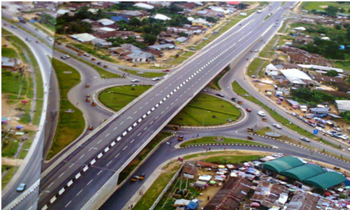
Fig. 1: Ariel view of Itam Bridge, Uyo, Akwa-Ibom (Source: Thisday Newspaper, 26 August, 2016).
