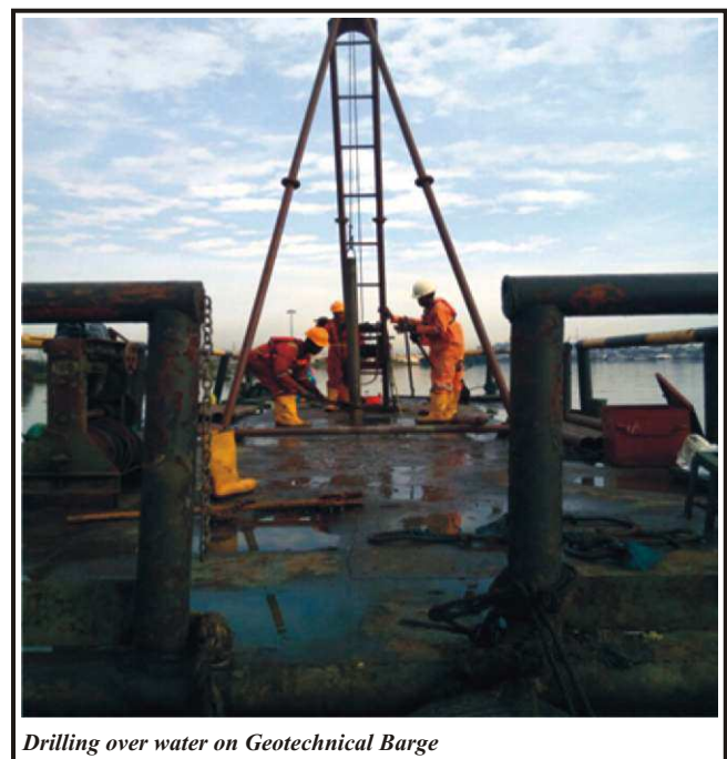
Fig. 1: Barge mounted rigs for geotechnical exploration
